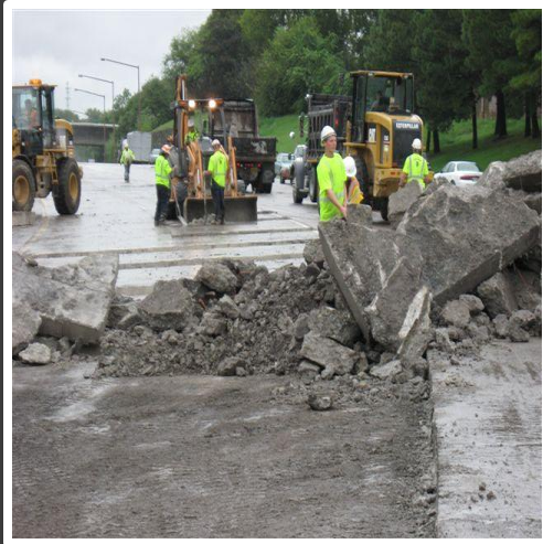
Damaged Concrete replacement
