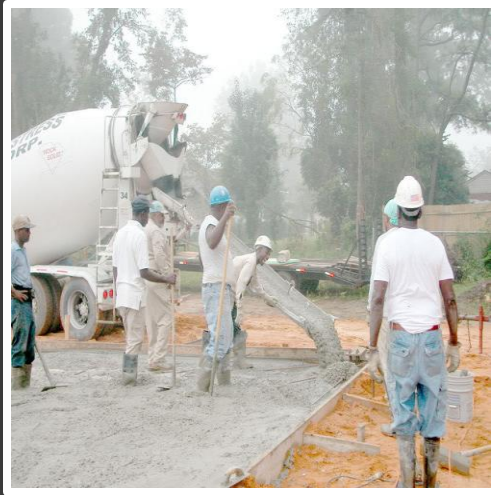
New concrete installation
